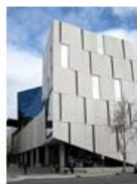
The Hawke Building, part of the UniSA, City West Campus.
